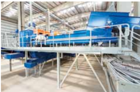
SORTING CENTER WASTES RECYCLING
