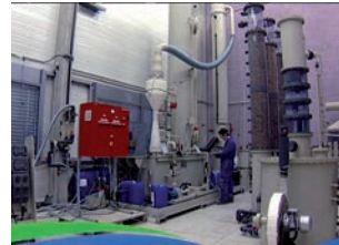
Pilot hall of more than 200 m 2
